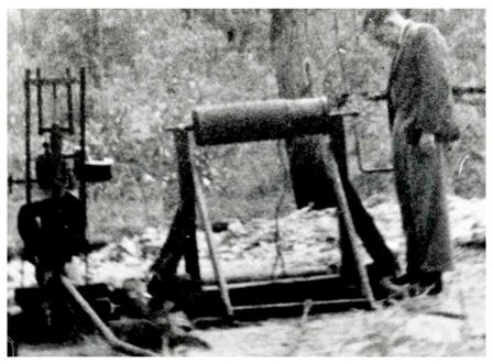
Buzzacott pump beside well being dug by hand. Note windless to pull up buckets of sand and gravel, as described by Roger Allen, May 1944. (Souwer family collection)
